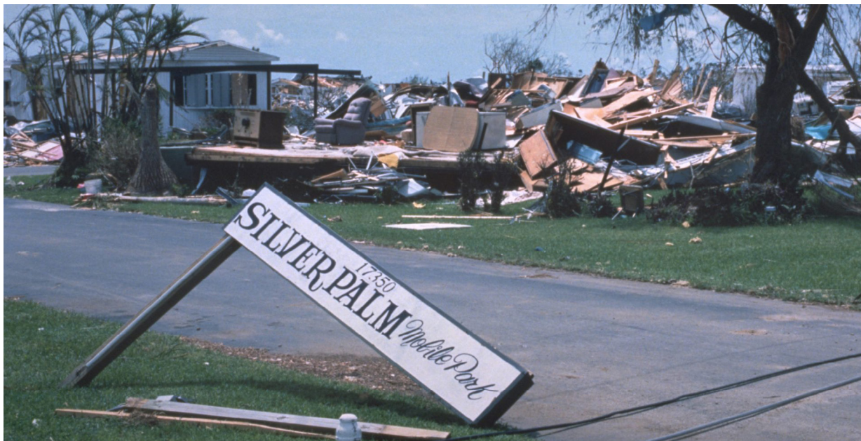
Silver Palm Mobile Park in Miami was devastated by Hurricane Andrew. After hurricanes, mobile home residents experience outsized losses and excessive cost burden compared to residents of multistory apartment buildings. Photo credit: Bob Epstein of FEMA News
